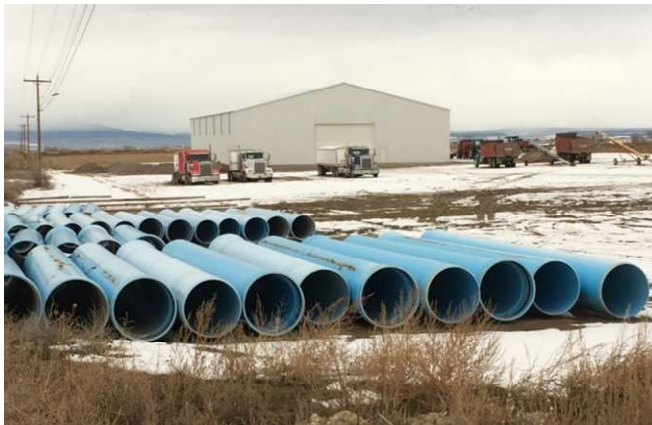
Figure 3 - Stockpile of PVC pipe used (left) used to enclose GB-GBA laterals (right) as part of Phase 9 East side lateral project of the Uncompahgre Project, north of Montrose, Colorado
