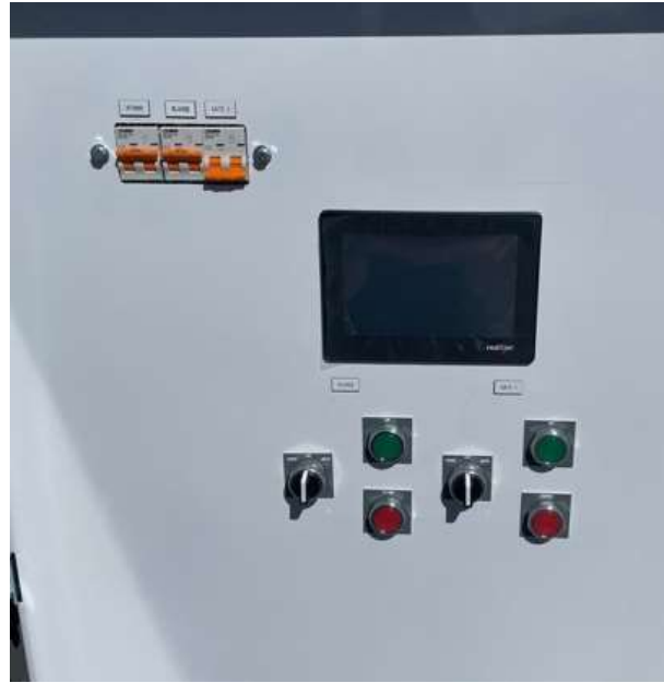
Figure 4 – SCADA controls installed at the Loutzenhizer Diversion, Uncompahgre River, south of Montrose, Colorado
