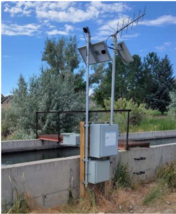
Figure 4 – SCADA controls installed at the Loutzenhizer Diversion, Uncompahgre River, south of Montrose, Colorado
