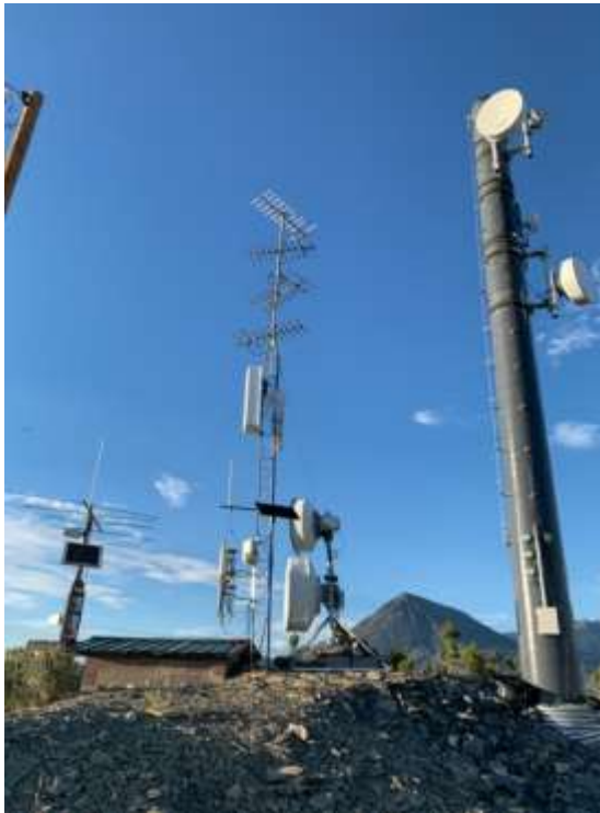
Figure 11 – SCADA network telemetry equipment installed on Young's Peak tower to assist with the transmission of regional information collected, Crawford, Colorado
