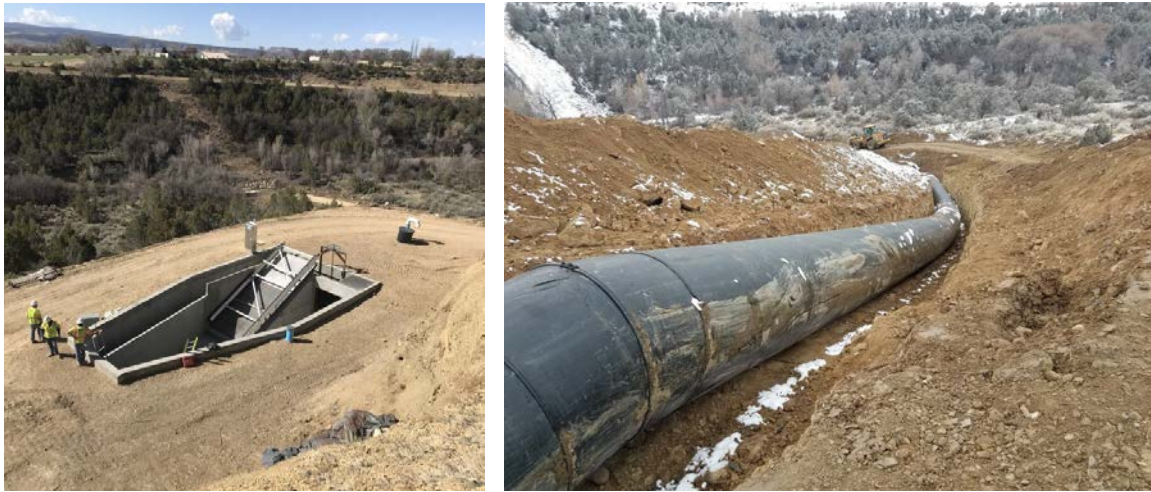
Figure 2 – Fire Mountain Canal Improvement Project: New siphon entrance and screen structure (left) with HDPE piping related to segment 47 pipeline (right)
