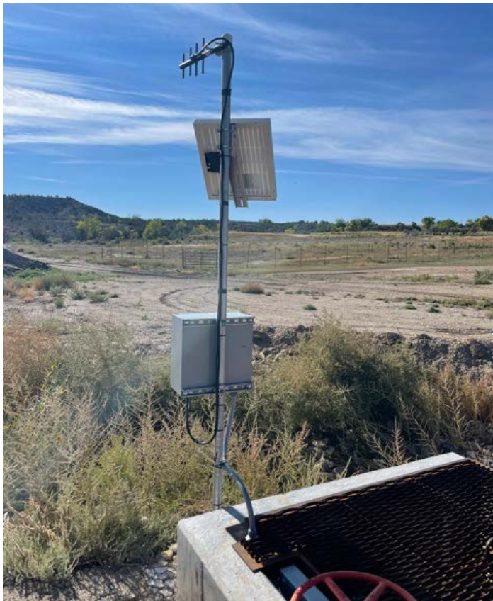
Figure 7 – Solar powered implemented SCADA system component at 4C regulating reservoir outflow, Crawford
