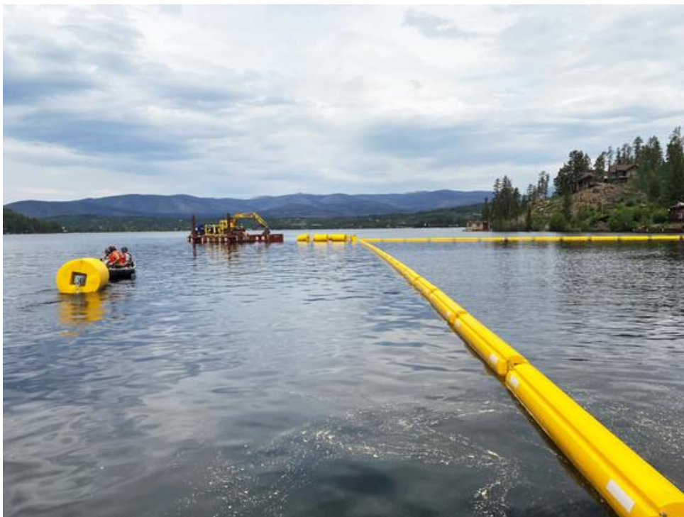
Figure 2. Debris boom installation at West Portal Adam's Tunnel. Courtesy of Northern Water.
