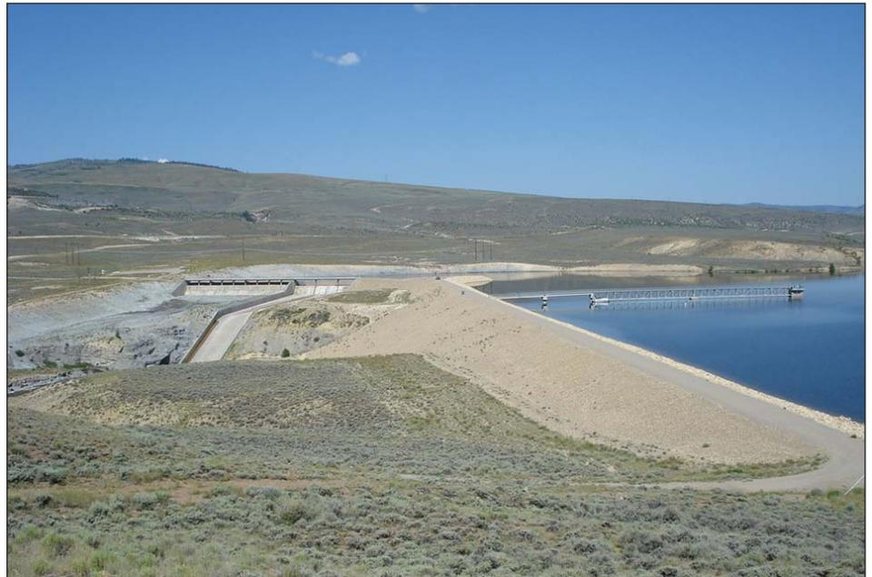
The crest of the Ritschard Dam at Wolford Mountain Reservoir will see construction work this summer to raise the crest to its originally designed elevation to make up for settlement that has occurred since the dam was put into operation in 1996. Despite a relatively poor snowpack year, the reservoir on Muddy Creek in Grand County is expected to fill by June 1, if not sooner.
